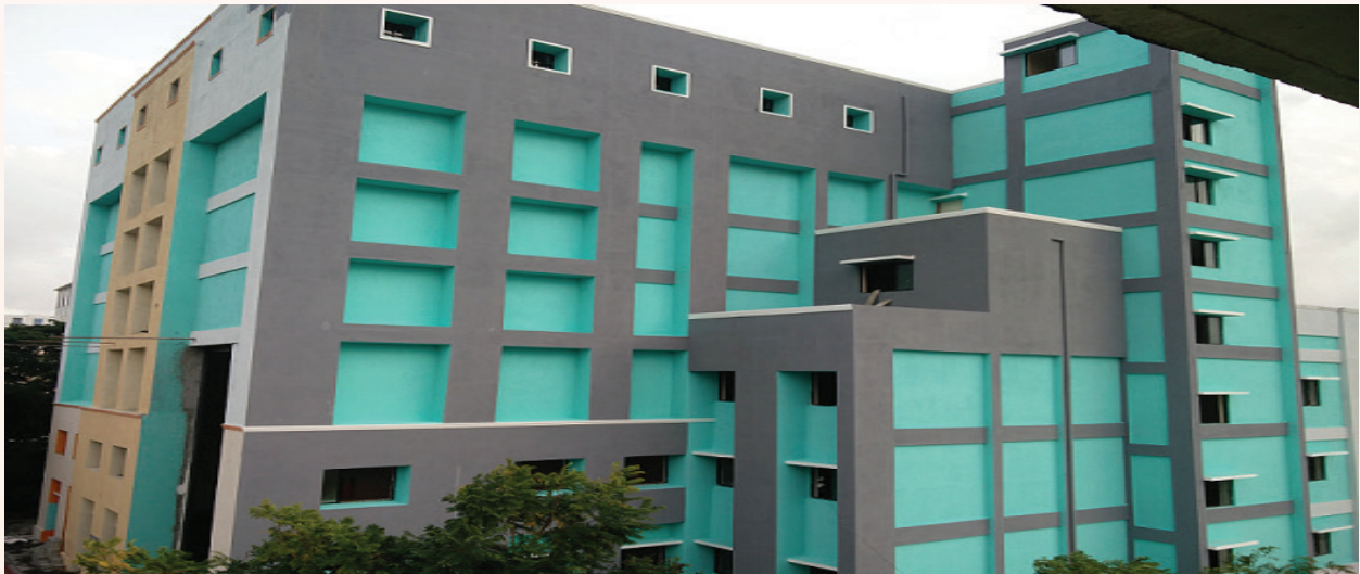
(Newly Constructed High Voltage Laboratory at NTH(SR), Chennai)
